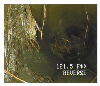
At the time of this report, it is unknown where the root blockage is in relation to the above exhibit. HDR is coordinating with the Contractor to obtain the location of their inlet numbering system and will provide an update on recommended actions at the Council Meeting.
