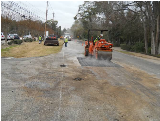
Rolling the asphalt repair in front of St Francis south bound lane. View to the north.
