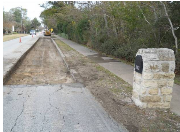
Asphalt repair on N. Piney Point between Shady Glen and Carsey Lane north bound lane. Removed the old Asphalt. View to the north.
