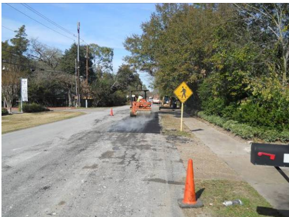
Rolling Asphalt between Shady Glen and Carsey Lane north bound lane. View to the north.
