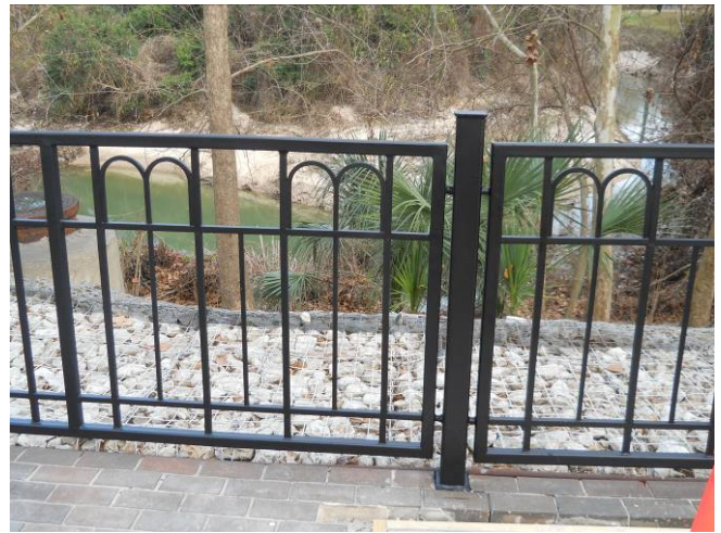
Repaired and repainted the metal fencing, panel # 1. View to the east.
