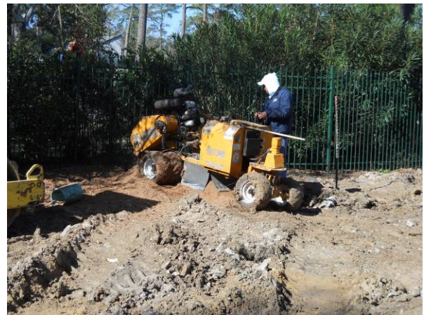
Performing stump grinding on Jan Kelly. View to the west.
