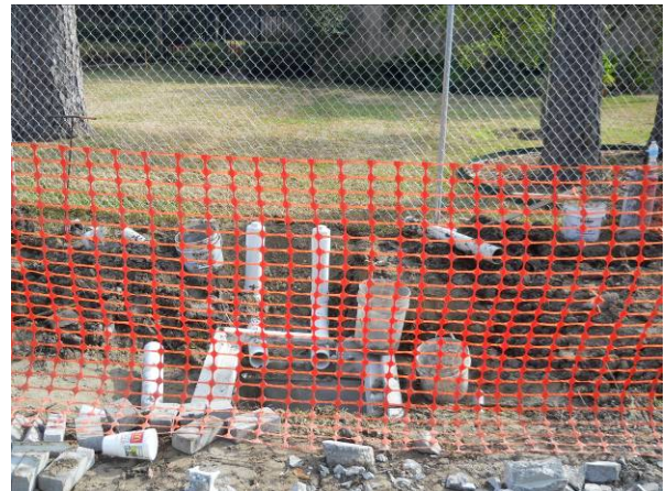
Install yard drains into inlet on the east side of Jan Kelly. View to the east.
