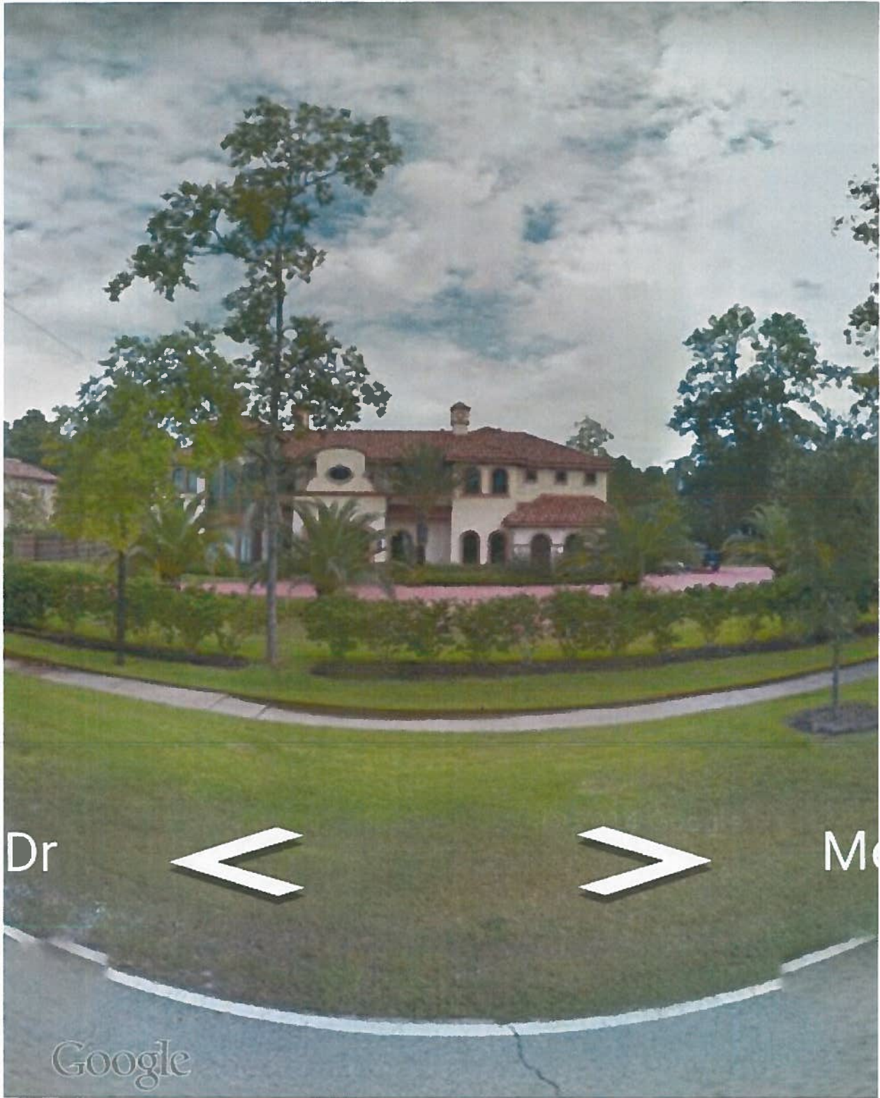
FIGURE 3-5: Pictures of the front of our property which shows vulnerability and easy access.
