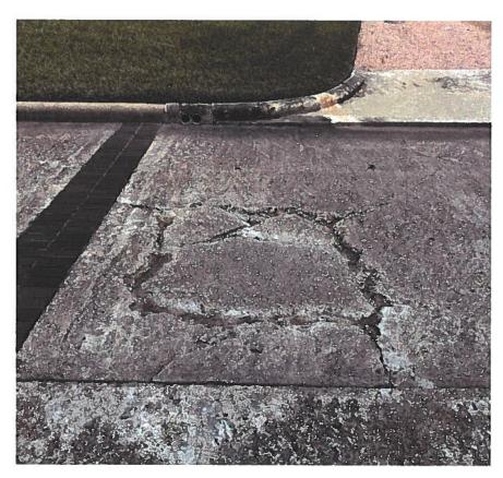
It is recommended that the full concrete panel be replaced. The Opinion of Probable Cost for concrete and curb removal, disposal, and replacement is approximately \$7,500.00. If approved, HDR will include the concrete point repair in the 2019 Maintenance Project
