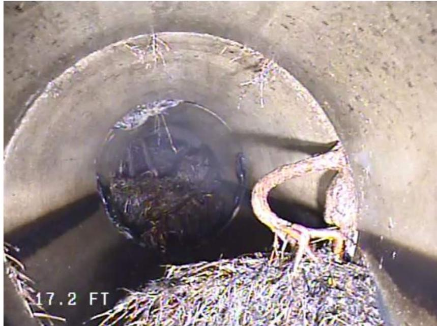
HDR contacted AAA Flexible pipe who completed the clean & TV work to obtain a quote to mechanically clean the roots out of the pipe. HDR will provide the quote to City Council for discussion upon receipt.
